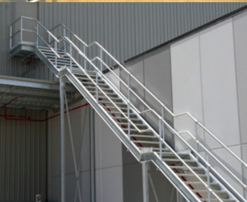
Installation - Type S2 Stairs & S3 Platform
