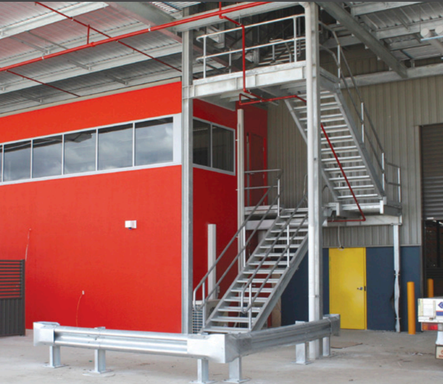
Installation - Type S2 Stairs & S3 Platform
